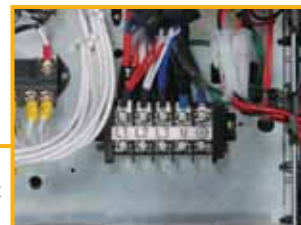
Outdoor unit power supply terminal block
