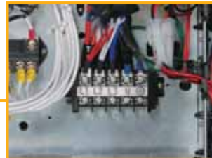
Outdoor unit power supply terminal block
